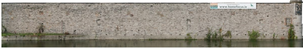
Figure 12.12: Riverside Stone Wall
