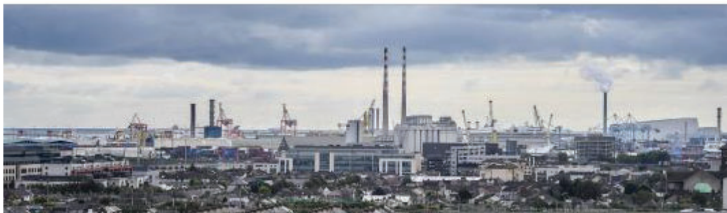
Figure 2.14: Guinness factory structure, Guinness Storehouse and Poolbeg Chimneys
