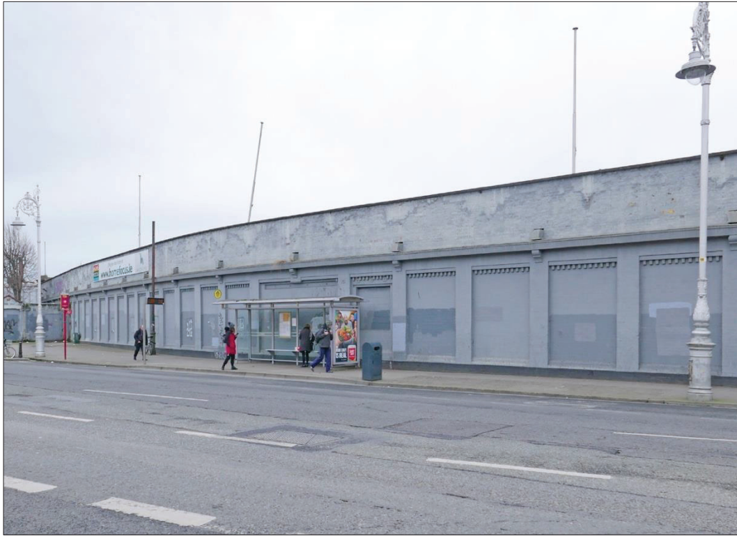
Figure 12.22: The long curved Wall of the Warehouse facing onto Parkgate Street
