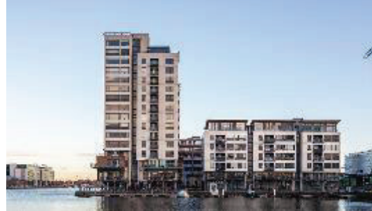
Figure 2.18: Millennium Tower – 67m
