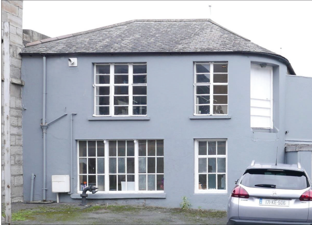
Figure 12.21: Two storey building attached to the inside of the arched entrance gateway
