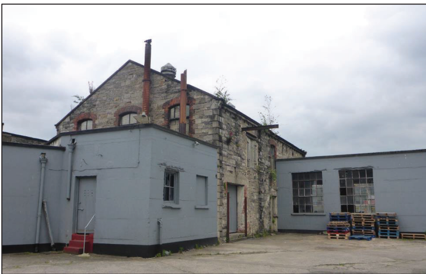
Figure 11.17: Late 19 th century gabled buildings viewed from interior of site
