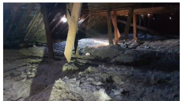
Figure 10.8: Attic space (B1)
